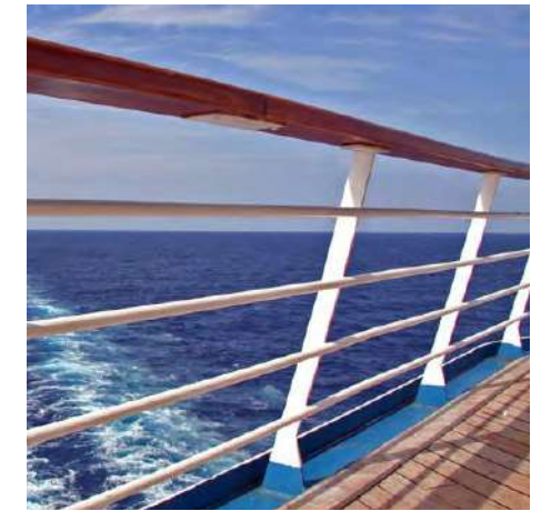
F10 -STAINLESS STEEL BALUSTRADE WITH TIMBER HAND RAIL
